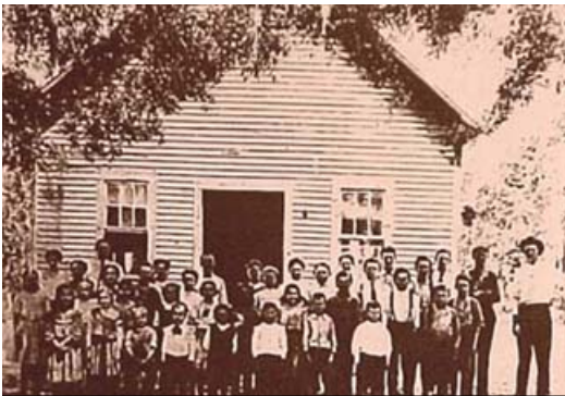
This is a picture of the first schoolhouse in Socrum. It was located just east of the present Bethel Baptist Church on the property of C. M. Witter, Sr., grandfather of R. Maloy. The building was also used as a Primitive Baptist Church on Sundays.
