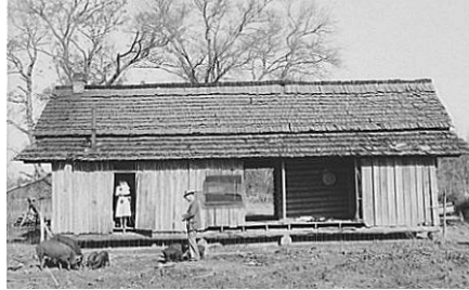
A dog-trot homestead, with the classic open breezeway between pens (Photo: Historic American Building Survey)
